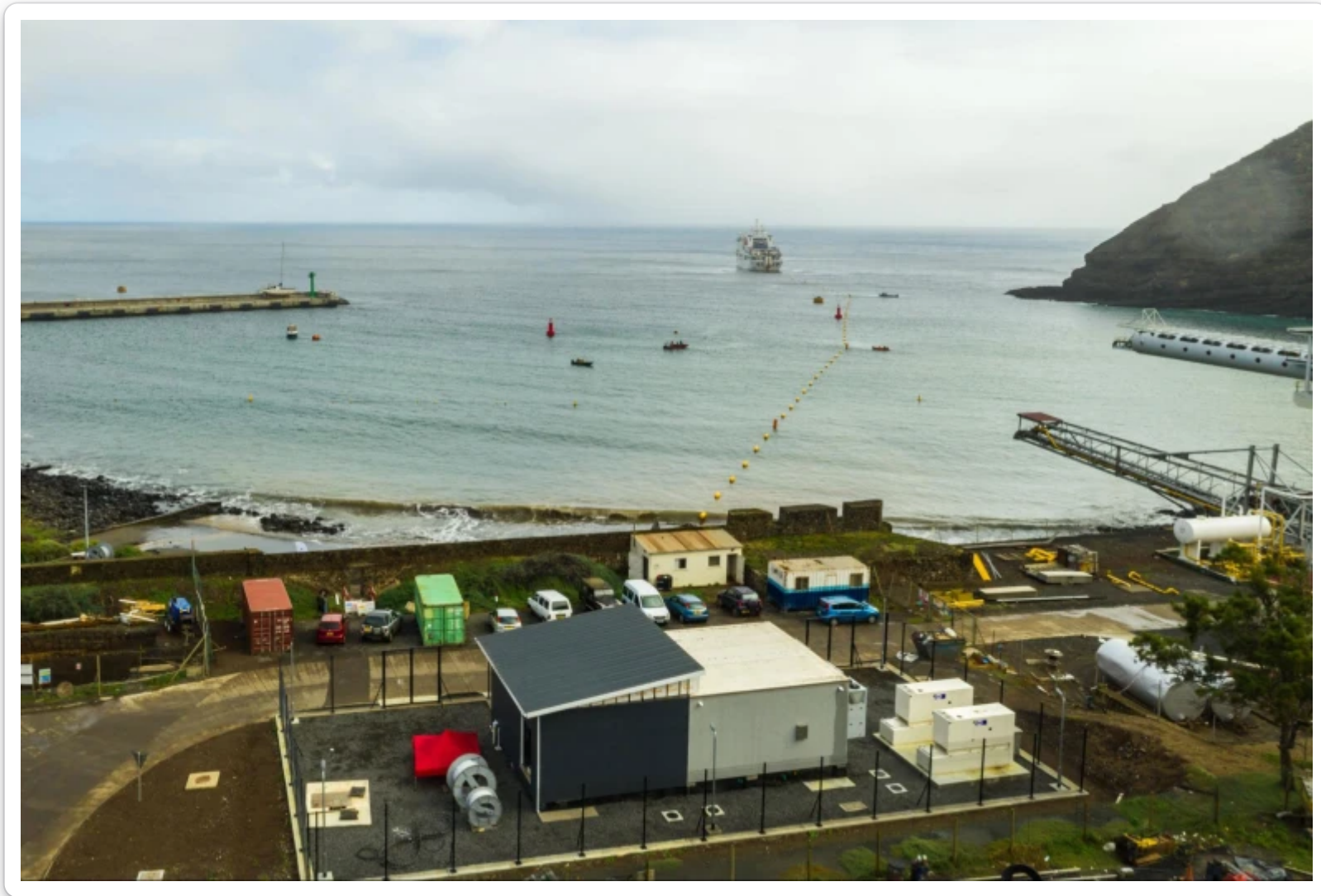
Landing of cable branch to the Equiano cable, August 2021
