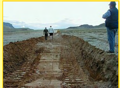
British Army Royal Engineers, working with Arup and Shelco specialists, supervise an investigative 'trial scrape' in July 2002, on the Prosperous Bay Plain site of the intended Temporary Construction-phase Airstrip. This will provide logistical support and an evacuation capability to the works contractor until the main airport runways are built and useable.
